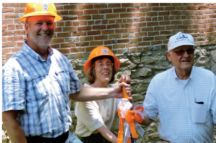
RIGHT: Corey Thomas of Pishny Restoration Services, Marion Smith of Engine House No. 1, and FAR President Tom Hall break ground on the Jeffris Project.
