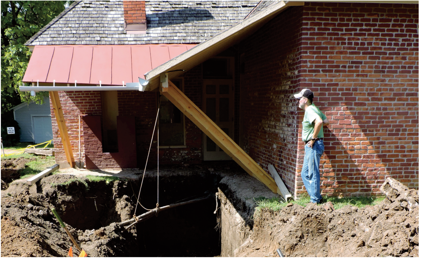
ABOVE: The crew dug out a cellar that had been loosely filled more than 50 years ago, but that was still holding water. LEFT: The ground around the Sites House is being regraded to better divert water from the building. BELOW: Marty Selby (center) visits with the project team following the groundbreaking ceremony.
